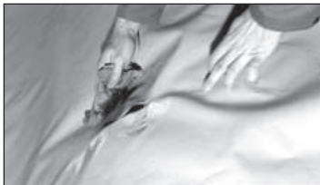
Washing of the duct textile around a tear.
