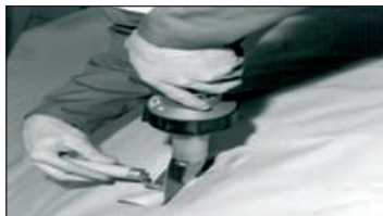
Hot-air welding of a patch seen from the outside .
