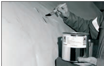
Application of adhesive.
