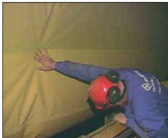
Inspection of duct.
