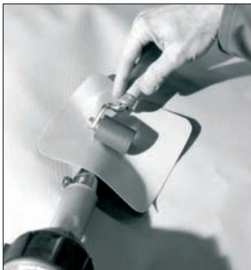
Hot-air welding of a patch and use of the pressure roller.
