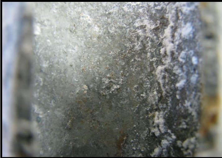
Photograph 17 showing the inner surface of Sample 1 after the 1000 hour exposure.
