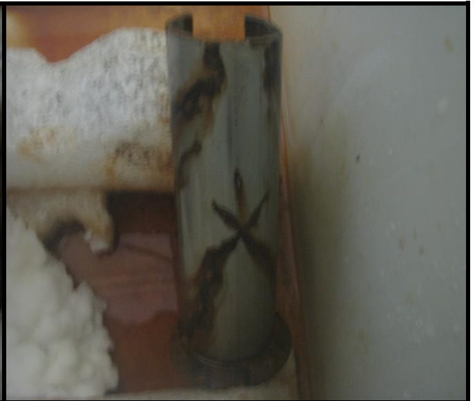
Photograph 36 showing the Sample 2 surface after 672 hours of continuous salt spray exposure.
