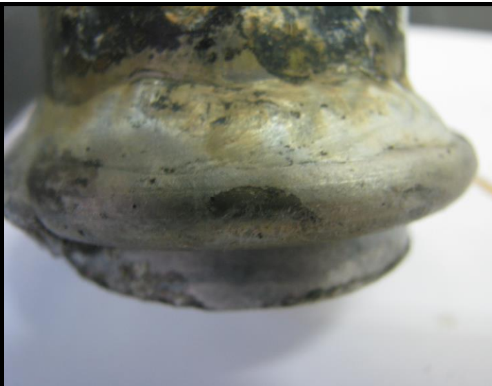
Photograph 21 showing the Sample 1 weld after mechanical and chemical cleansing.
