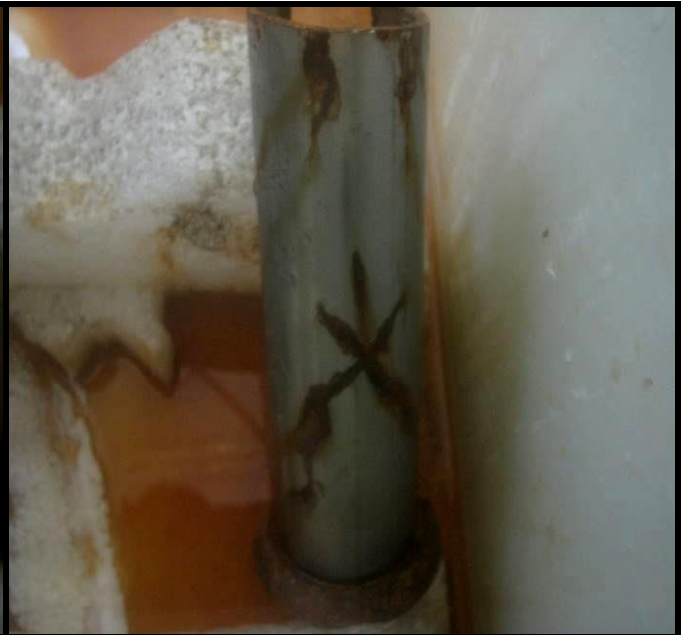
Photograph 28 showing the Sample 2 surface after 96 hours of continuous salt spray exposure.
