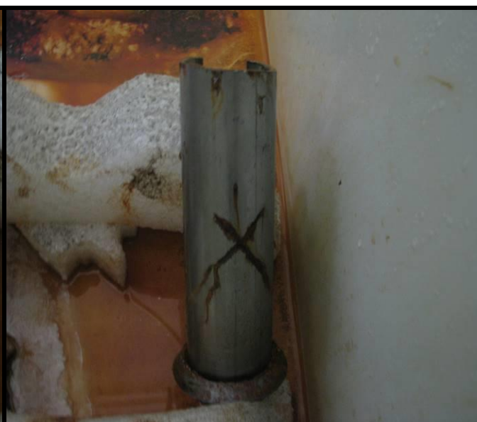
Photograph 24 showing the Sample 2 surface after 24 hours of continuous salt spray exposure.
