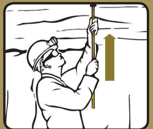
8 Remove cable from hole, turn it around and remove pipe sleeving from mechanical shell. Insert the cable right-way-up to end of the hole.
