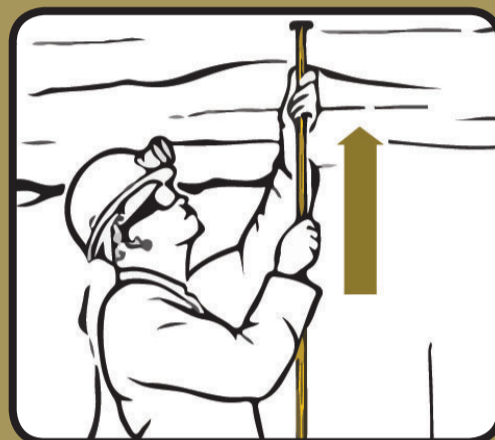
7 Remove face plate, sponge, barrel and wedge components. Insert cable upside-down into hole, to measure depth. If hole is not deep enough, re-drill hole to required depth.
